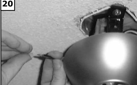
Make wire connections to power source using wire nuts provided. Make sure that no filaments are outside of the wirenut. After making the wire connections, the wires should be spread apart with the grounded conductor and the equipment-grounding conductor on one side of the outlet box and ungrounded conductor on the other side of the outlet box.
